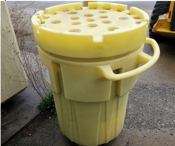
Spill kit is in the open. Could be covered or indoors (if accessible).
