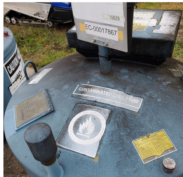
Signage covered in soot. Has WHMIS 1988 symbol (old symbol, incorrect – should be TDG). Take off old symbol, clean and ensure visible signage.
