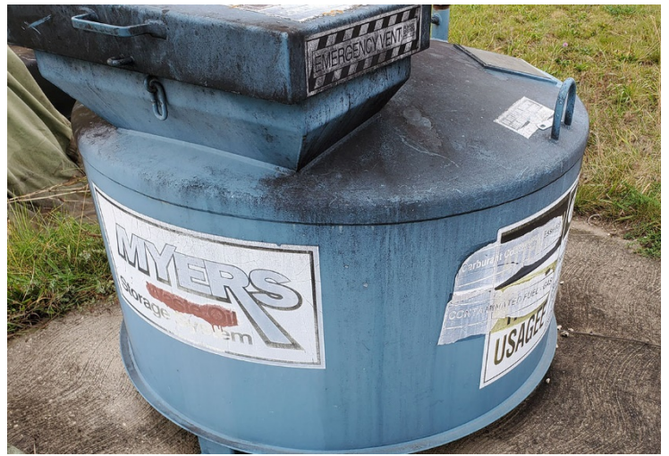
Waste oil is stroked out – remove and affix appropriate signage.
