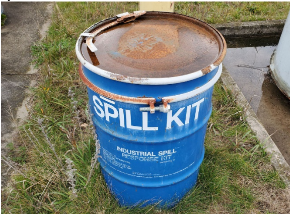
Spill kit is sitting outside and rusting. Place tank in an accessible building or at least under cover.
