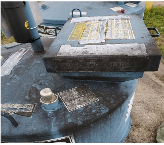
Various signage. Covered in soot. Remove soot. Correct signs only.
