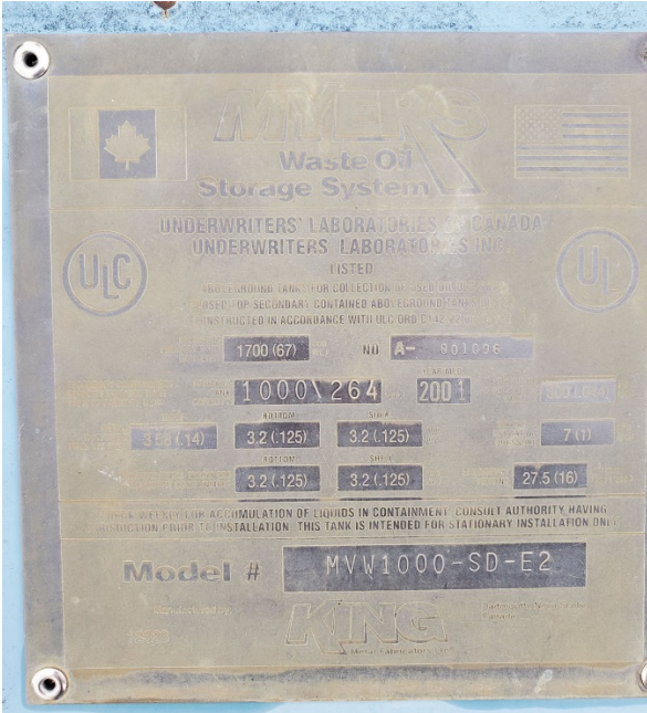
Certification is for waste oil only – have gas, diesel and antifreeze.
