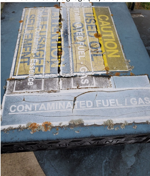
Lots of faded signage over used oil sign. Remove incorrect signage and place new signage.
