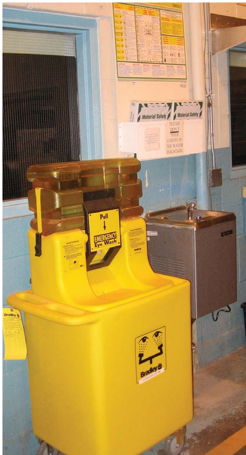
Portable eyewash stations can provide improved response due to their mobility and still provide 15 minutes of continuous flow treatment.
